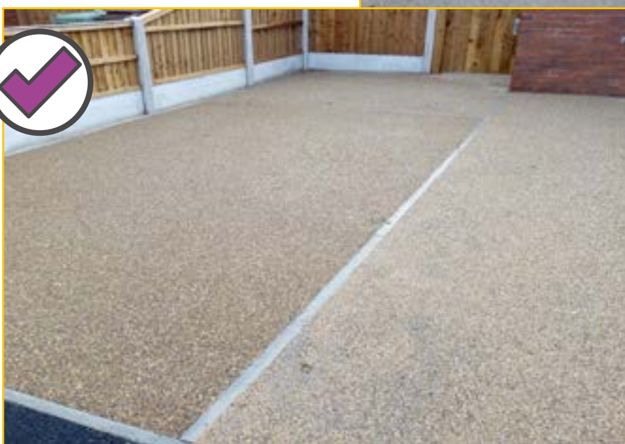
Permeable resin drive
