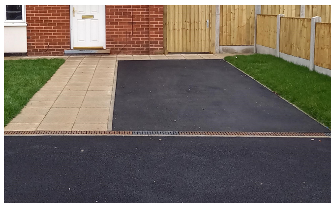
WDH Environmental scheme approved driveway (drainage channel to front)
