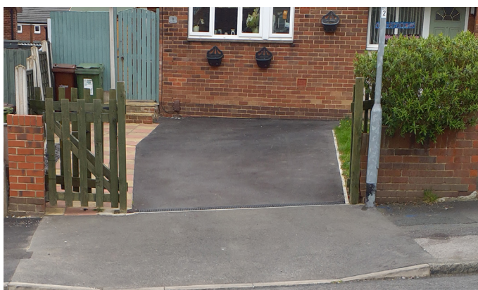
Tenant approved driveway (drainage channel to front)
