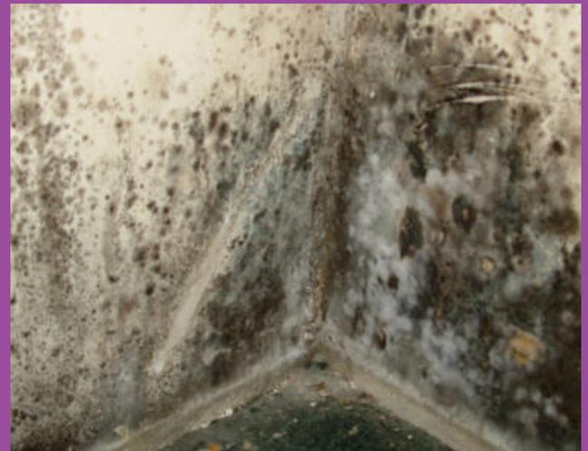
This mould only grows in the pure water produced by condensation and although black mould is the most common, mould can be many colours when growing on other surfaces such as carpets, curtains, bedding and clothing.
