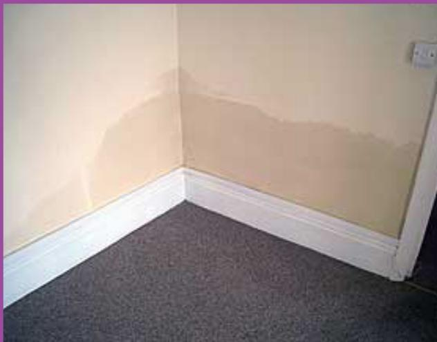
Rising damp from floor level before plaster damage has taken place.
