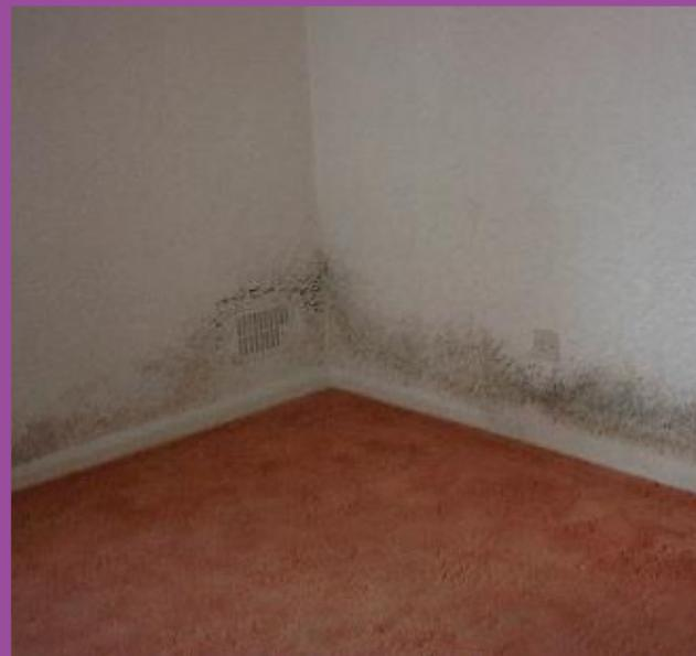
This picture shows extensive black mould growth at low level indicating poor ventilation and air circulation.
